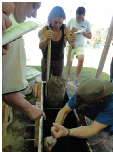
ramming the prepared earth
