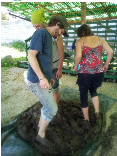
Preparing the mixture for the plastering
