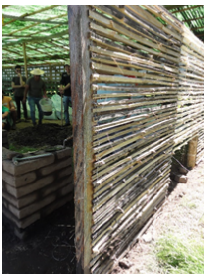
Structure ready to receive the mixture
