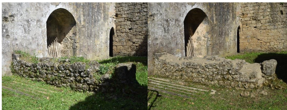
Before / After the masonry work
